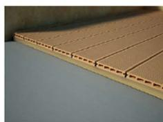
Ensure the deck is cut square in both the vertical and horizontal plane to enable the boards to locate accurately and create a neat joint.
