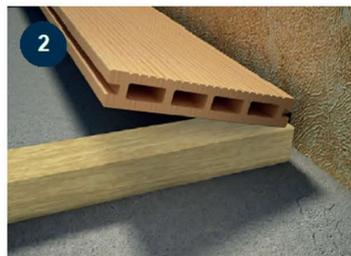
Tilt the first decking board so the leg of the deck clip locates underneath the lip of the starter clip.
