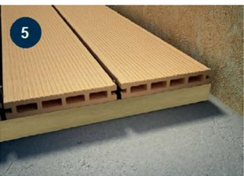
Once the next board is pushed into place at this point tighten the screw while applying a little horizontal pressure to the new decking board.
