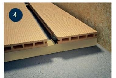
Fix the deck clip with the screw. Do not over tighten the screw as this makes it difficult to locate the next board.
