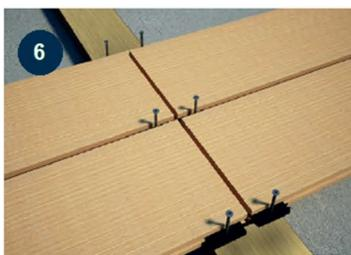
A double bearer (joist) is required when joining decking boards
